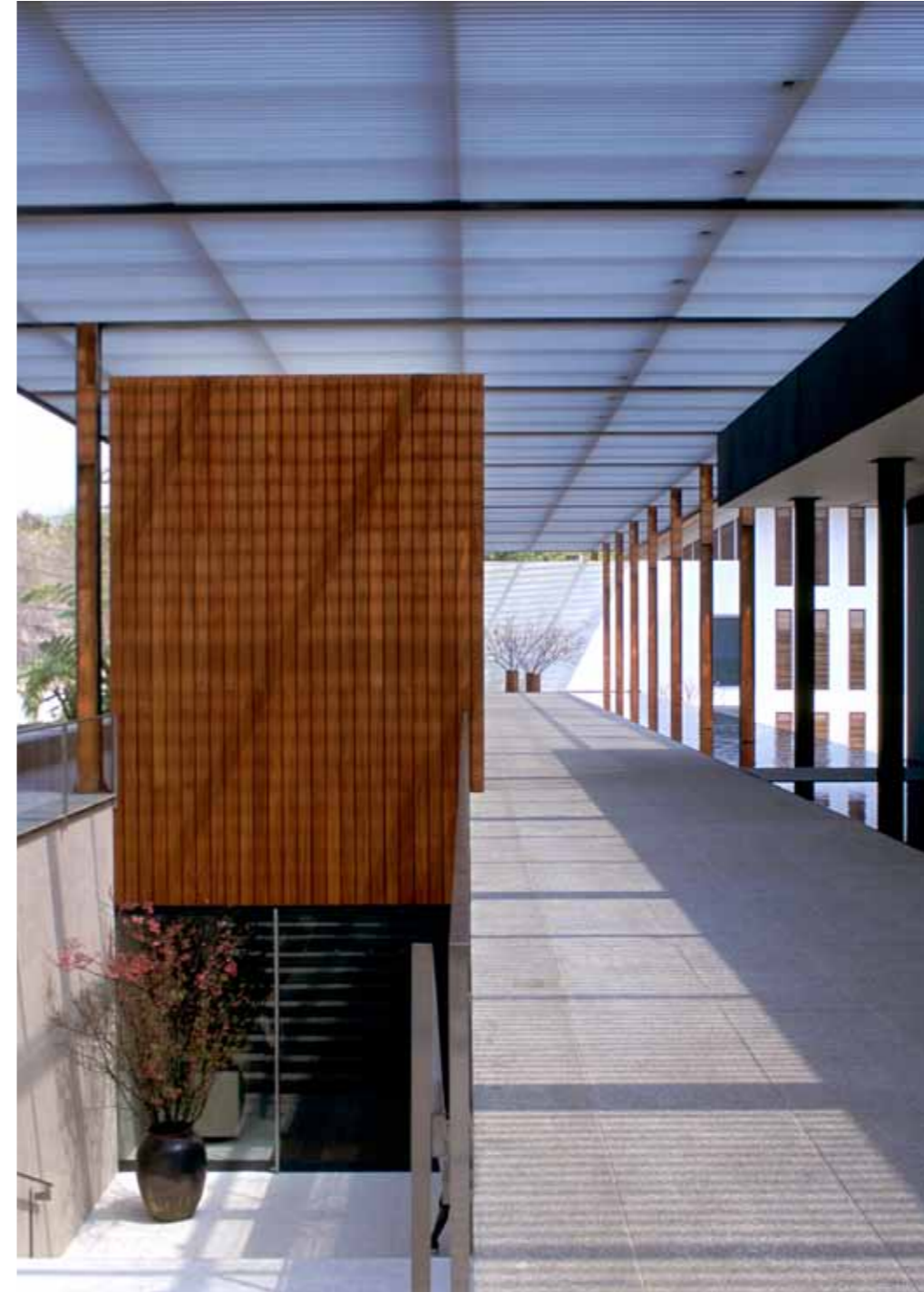
This page, left: The retail space is a timber-clad box, inserted into the arrival concourse. Right: The arrival area is a balanced juxtaposition of timber, stone and glass elements.
