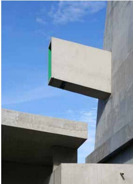
The west light canon, right over the entrance to the church.
