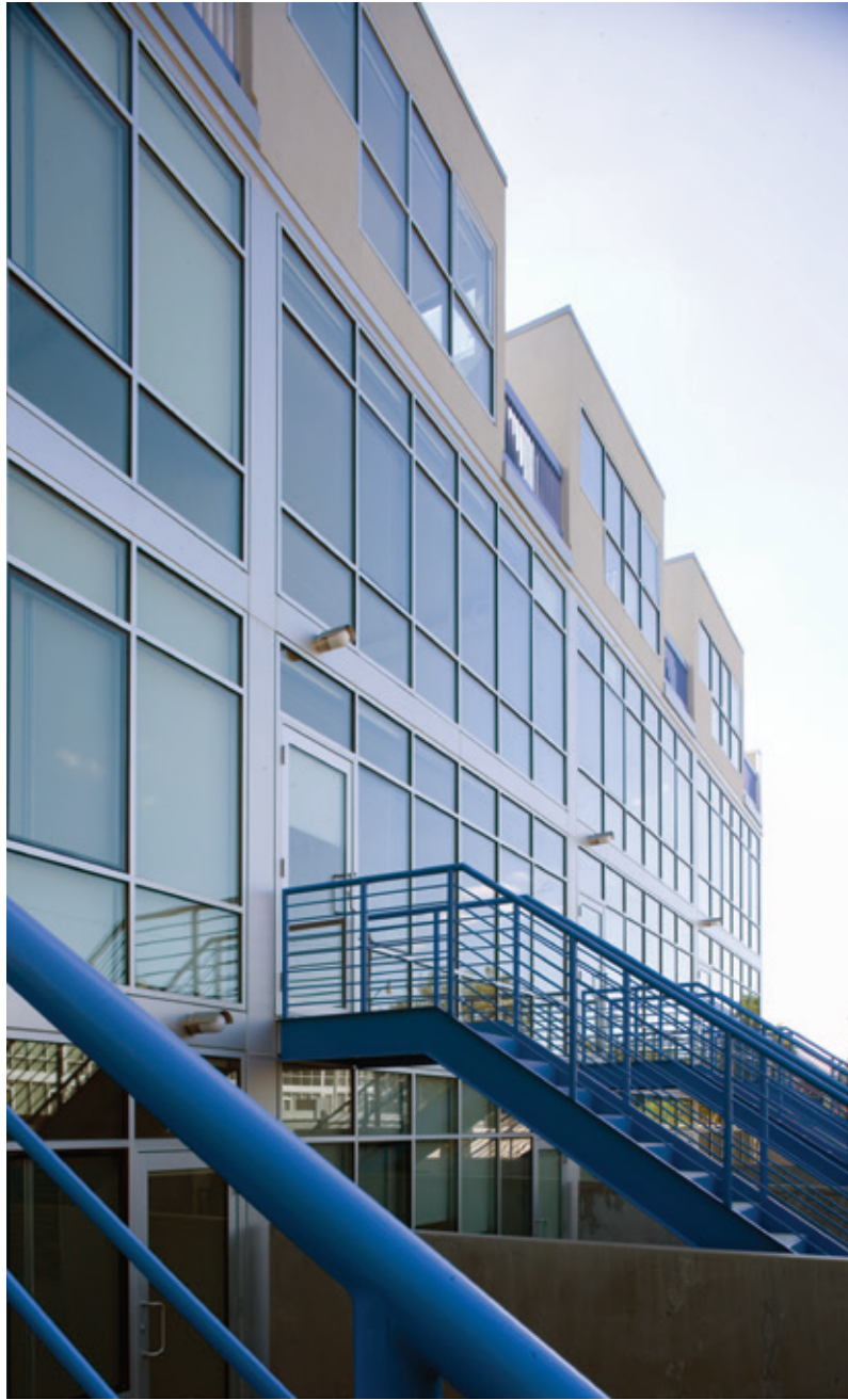
LEFT North façade with private entrances to each unit from parking BELOW Section RIGHT Upper unit master bedroom
