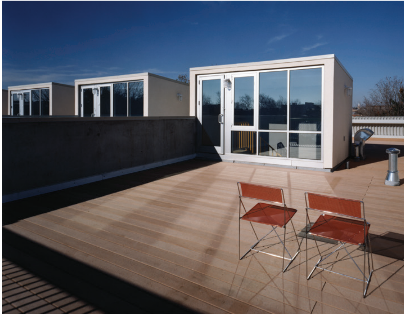
ABOVE Top unit private roof deck RIGHT Alley façade with parking
