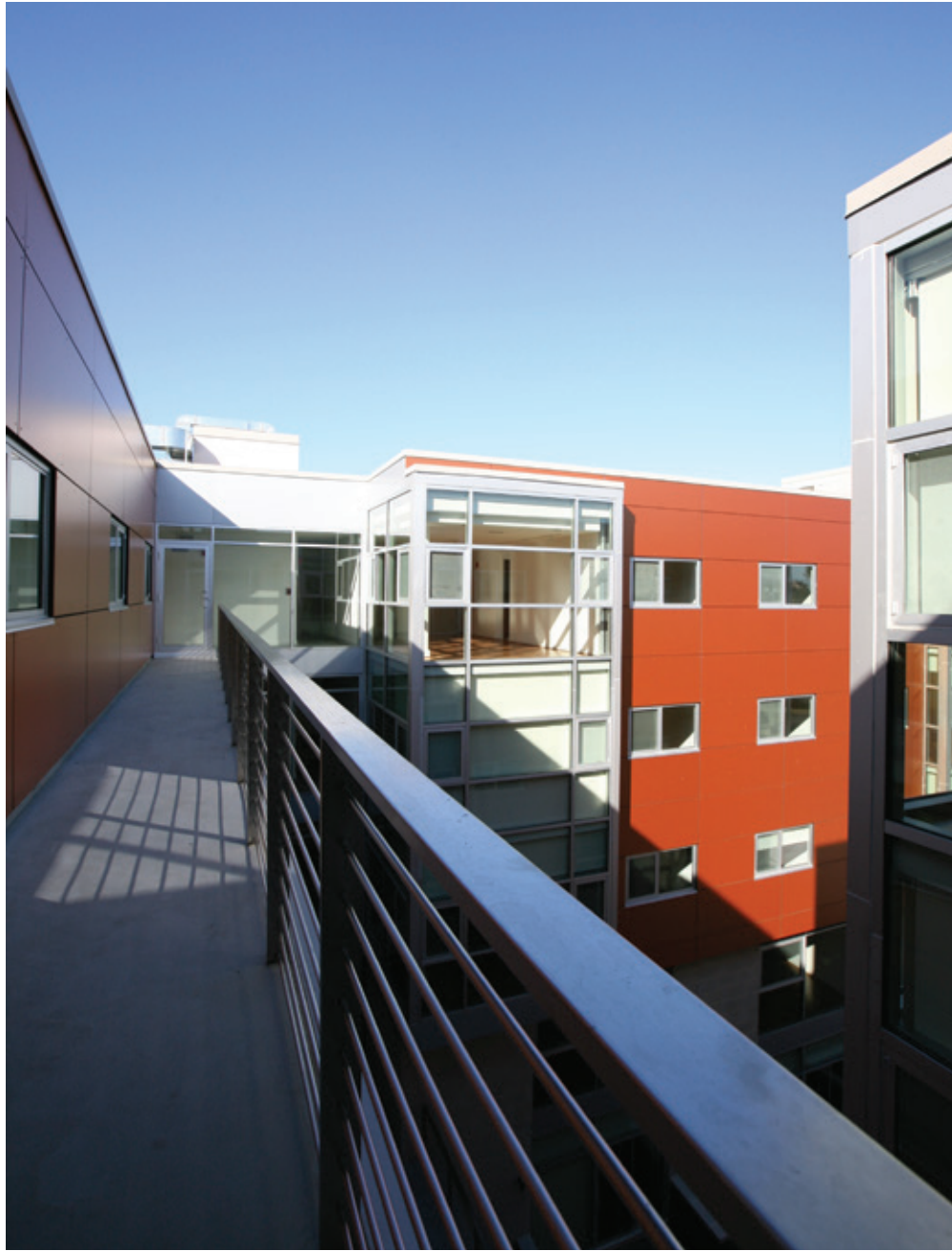
LEFT "Outdoor hallway" as means of a second exit RIGHT Typical unit living space
